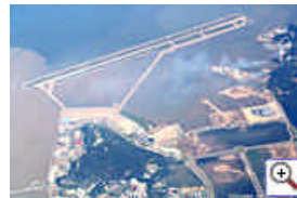
Macau International Airport
