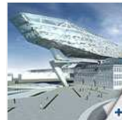
Havenhuis Antwerpen (work in progress) Studeburo Guy Mouton
